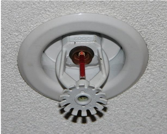
FIGURE 4.1 Bulb sprinkler head.
